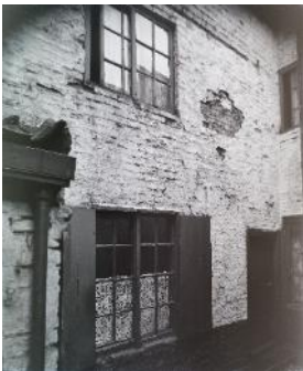
Burn's Entry Perished brickwork to rear of Burn's Entry, Market Place. 1 item
